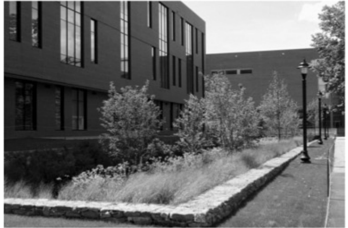
This large sunken vegetated area is a “bioretention” LID practice that processes the runoff from a large roof on the UCONN campus.
